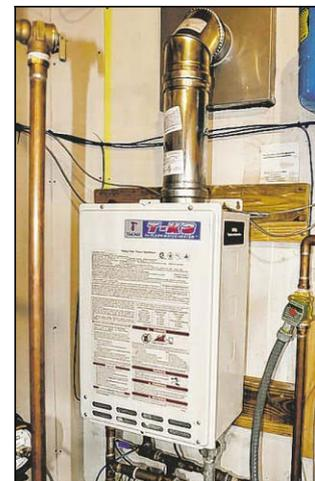
cient than standard electric water heater. Doesn't have the standby energy losses associated with water heaters that store water, which can save you money.
