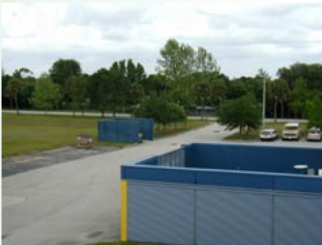
Figure 7. The blue enclosure in the background allows trash dumpsters to be kept away from the facility.
