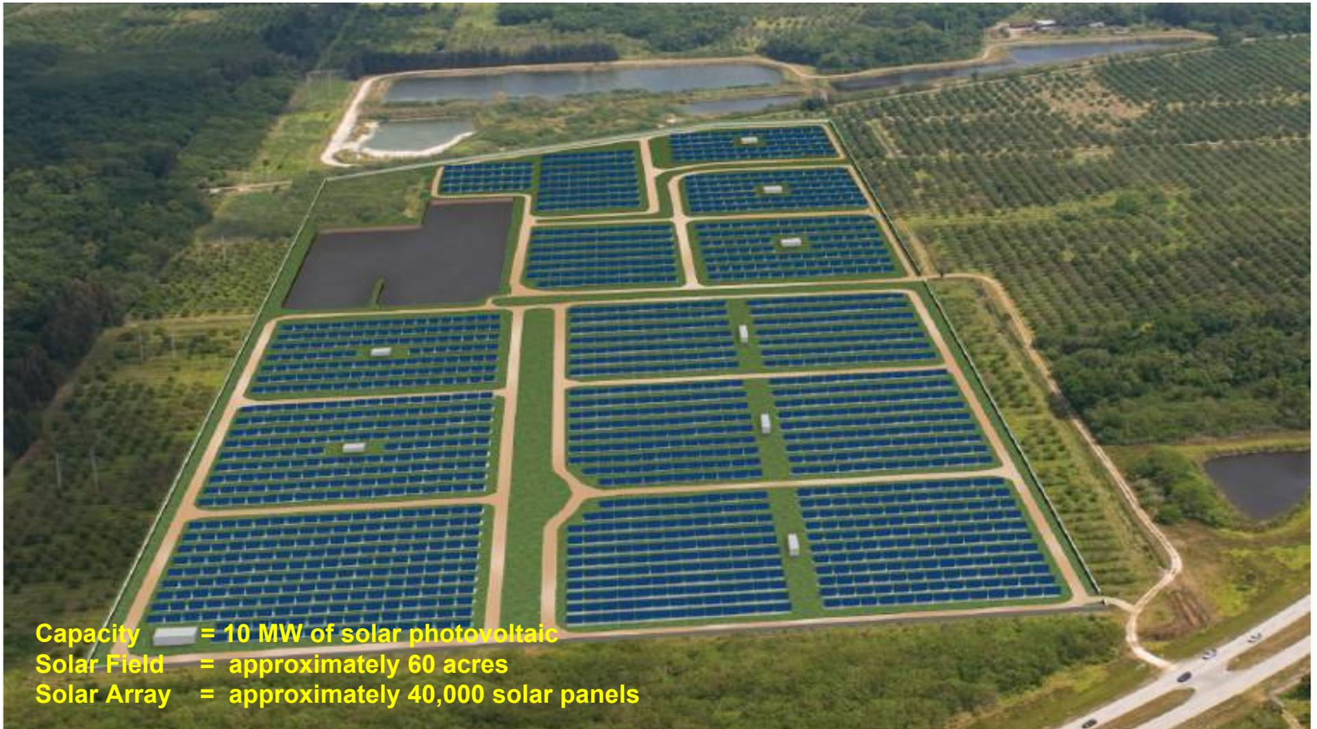
**Capacity** = 10 MW of solar photovoltaic
