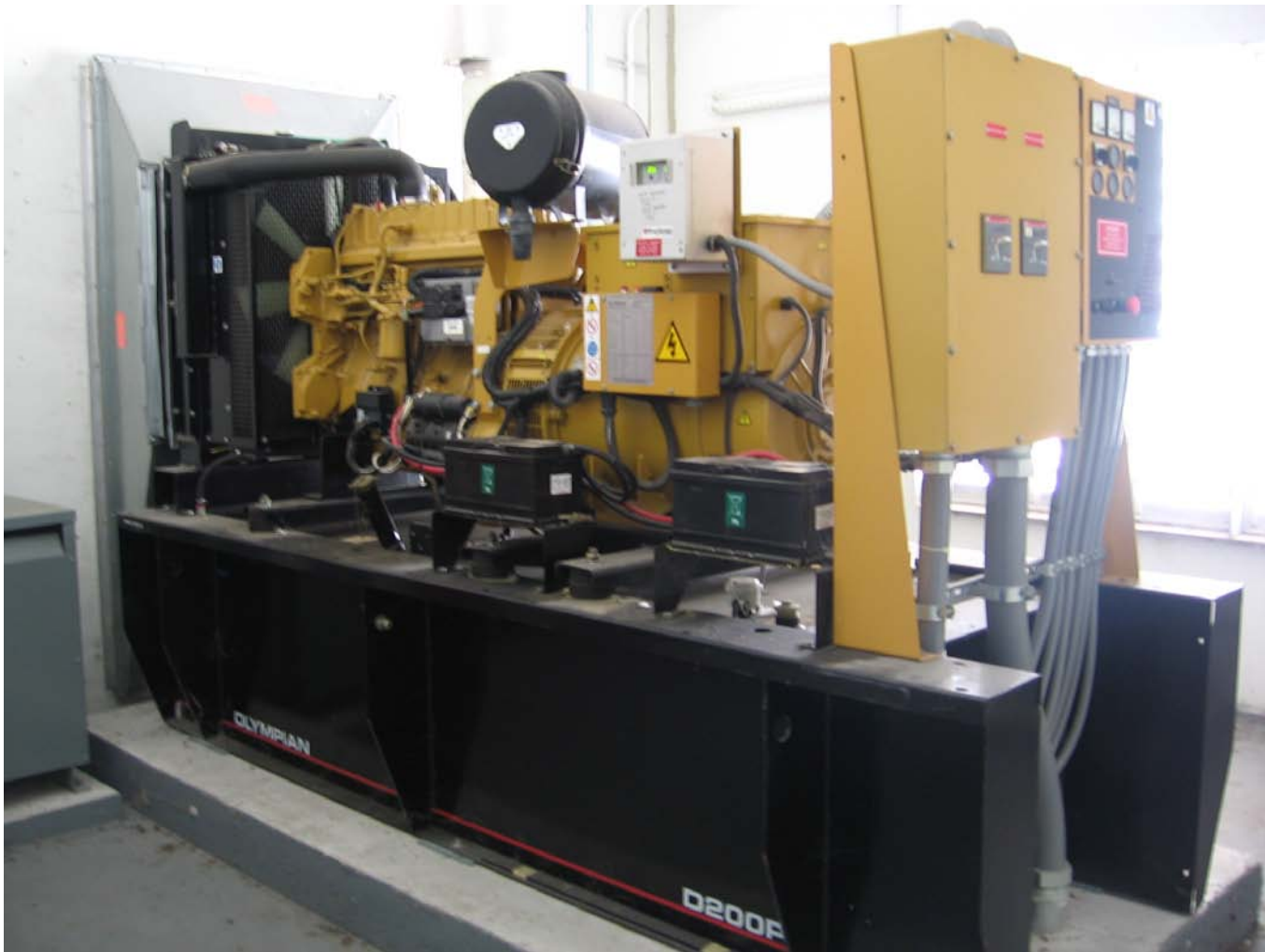
Olympian D200P3 200kW stand By generator set
