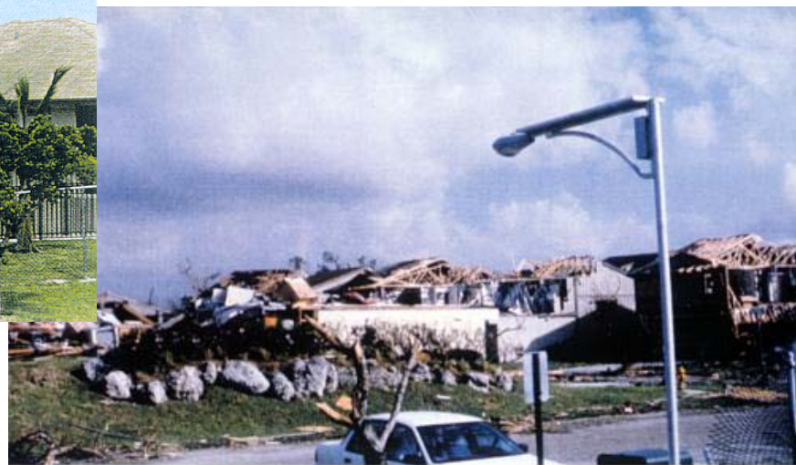
After Hurricane Andrew, Picture facing N.W.
