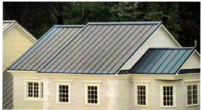
Figure 11. This is an example of a building that integrates flexible PV laminates and conventional metal roofing. (Photo courtesy of United Solar Systems Corporation.)
