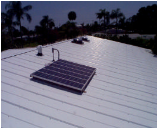
Figure 9. Conventional stand-off arrays mounted on metal roofs may have lower life cycle costs than almost any other array-roof configuration.
