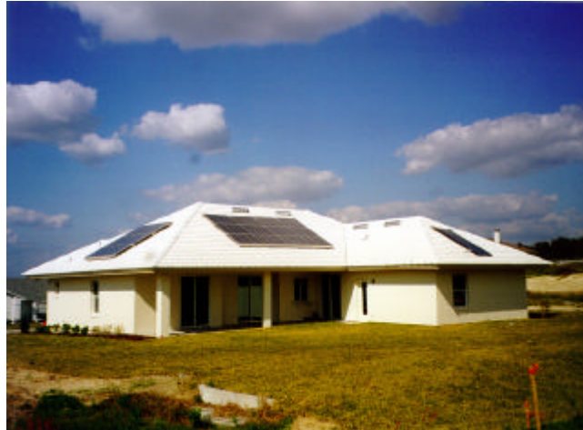
Figure 5. This PV residence in Lakeland combines the best in building energy and photovoltaic technologies.
