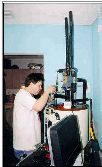
Figure 6.3-3. Working in restricted areas.
