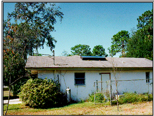
Figure 6.3-4b. Unshaded collector provides solar gain throughout the day.
