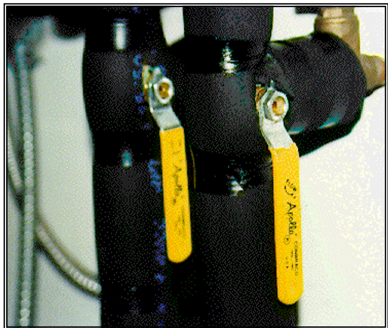
Figure 6.3-16b. Excellent insulation installation.
