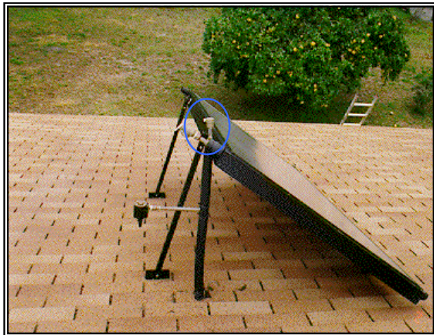
Figure 6.3-12b. Air vent installed in true vertical position.
