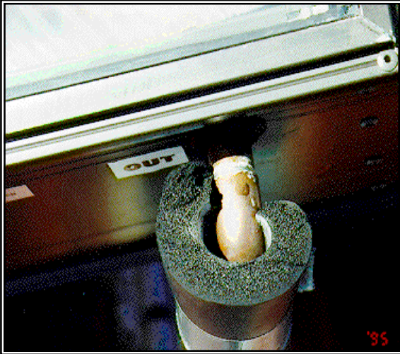
Figure 6.3-11a. Ends of pipe runs should be well butted.
