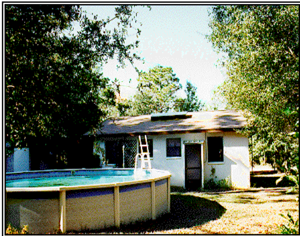
Figure 6.3-4a. Collector is shaded during much of the day.
