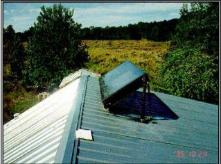
Figure 2.1-1. ICS system installed on a rural residence in North Florida.
