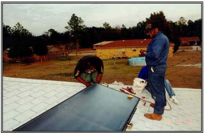
Figure 2.1-3. Local plumber installing ICS system.
