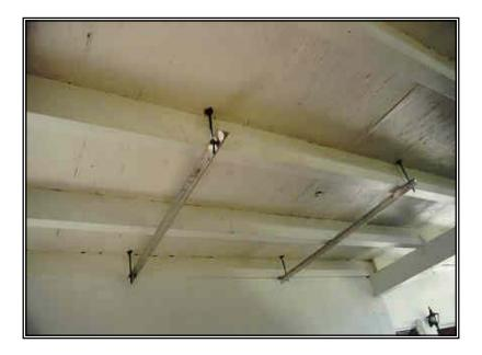
Figure 2.2-2. Spanner mounting of solar collector.
