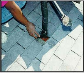
Figure 2.3-3. Standard solar industry flashing.
