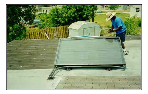
Figure 2.3-6. Twenty-five-square-foot collector installed on Miami site.
