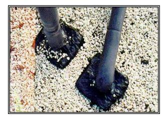
Figure 2.3-1. Pitch pan filled with bitumen.
