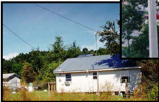
Solar system installed on country home in rural North Florida.
