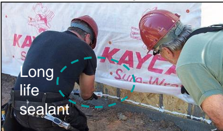
Seal air barrier at edges and seams
