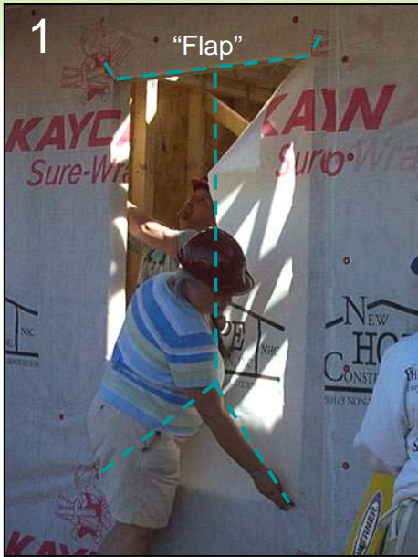
1 Cutting “Modified I” or “Inverted Y” opening in house wrap
