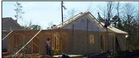
House wrap applied to gable end before raising truss into place
