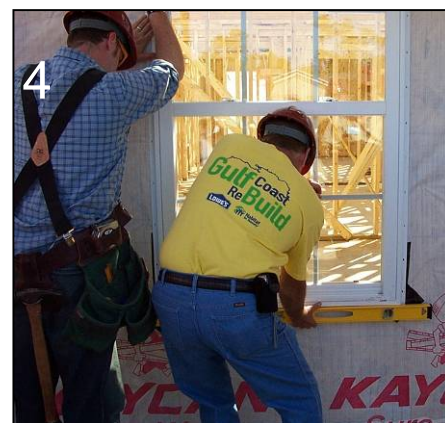
4 Set window, pressing to set sealant against house wrap
