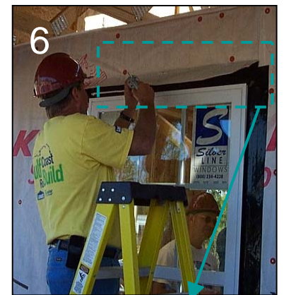
5 Shiplap side flashing over nailing flange and sill flashing, under house wrap “flap”
