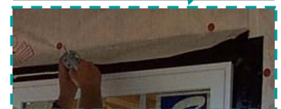
6 Long life sealant under flap
