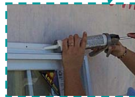
Apply long life sealant to back of nailing flange
