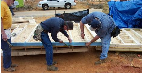
Sill seal – keeps air and bugs out
