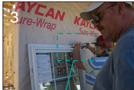
Apply long life sealant to back of nailing flange
