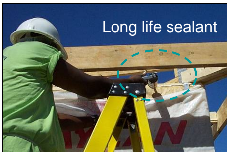
Seal air barrier at edges and seams
