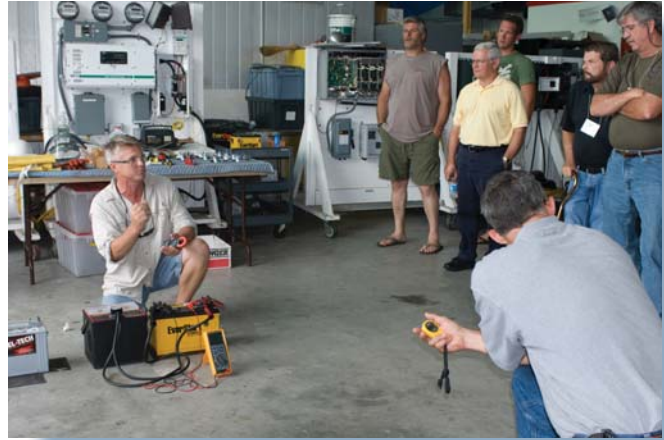
Photovoltaics course instructor, Donard Metzger, provides instruction on how to test a battery's load.
