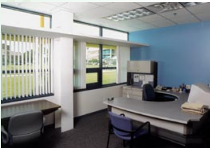
Figure 8. In this office, desks are positioned to take advantage of available daylight. Light shelves extend horizontally from the windows and help diffuse the natural light and control glare, as do interior blinds.
