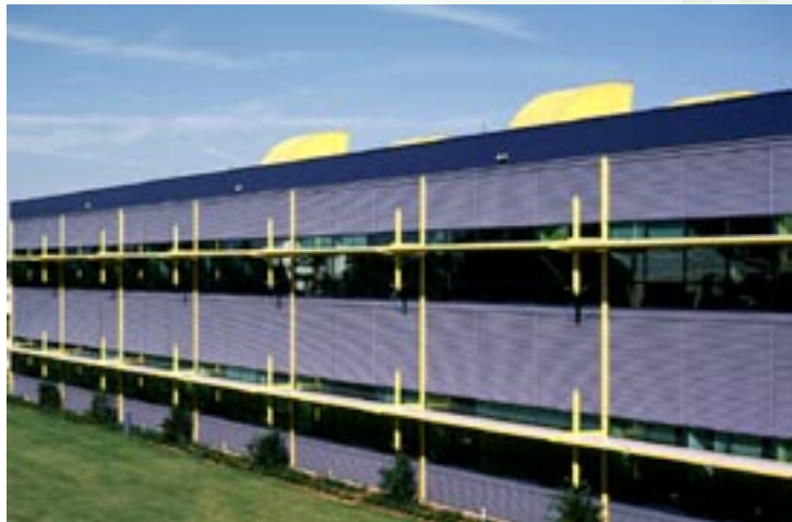
Figure 19. Window shading devices can be incorporated into the architecture of a building, such as these exterior light shelves at the Florida Solar Energy Center in Cocoa.
