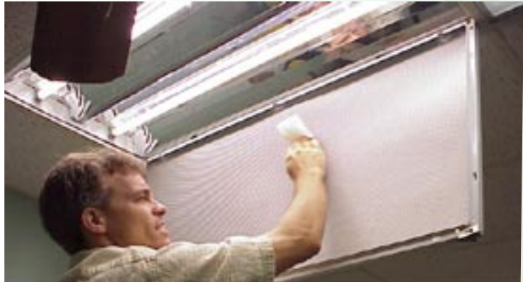
Figure 16. Regular fixture cleaning is an important part of a planned lighting maintenance program.
