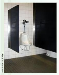
Figure 23. Stalls and partitions should be suspended from the ceiling or extend from a wall to permit easy floor mopping and reduce build-up of soil on legs and other floor supports.
