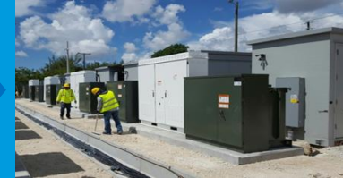
1.5 MW / 4 MWh using 2 nd life EV Batteries
