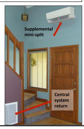
Key Takeaway: Runtime of a low efficiency existing central system can be offset with a high efficiency supplemental system. Supplemental system provides redundancy if central system fails.
