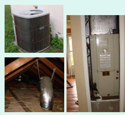
SEER 8.7, HSPF 6.75 Heat Pump with better than typical duct leakage (qn,out = 0.05)
