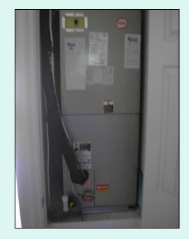
Closet gutted, drywalled; new return plenum & platform constructed
