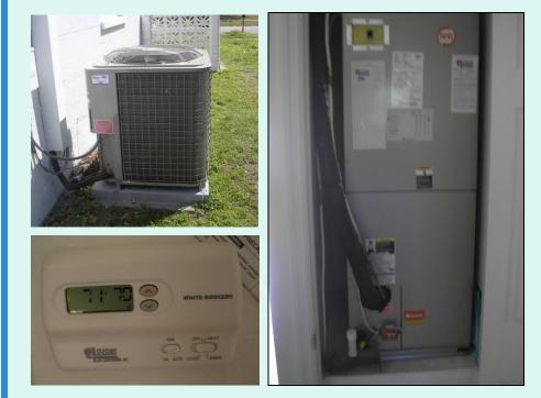
SEER 15, HSPF 8.8 Heat Pump with sealed ducts (qn,out = 0.02)
