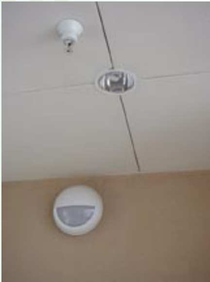
Figure 17. Light fixtures that direct light downward, where it is needed, minimize light trespass.
