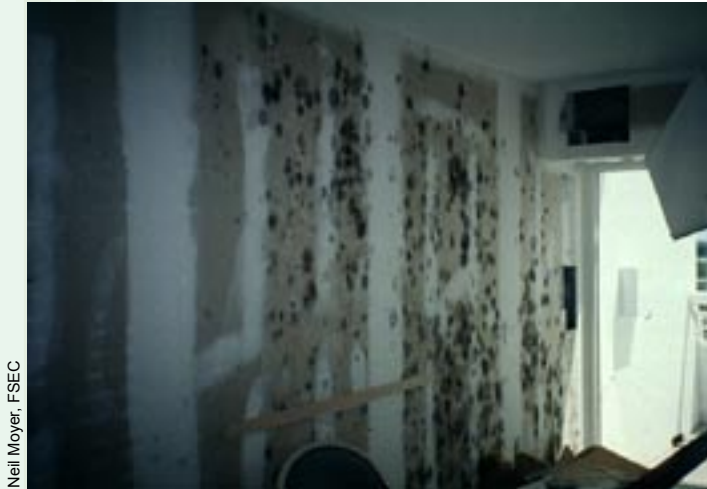
Figure 6. Water can enter a building envelope in the vapor form, and become trapped behind an impermeable barrier, such as vinyl wallpaper.
