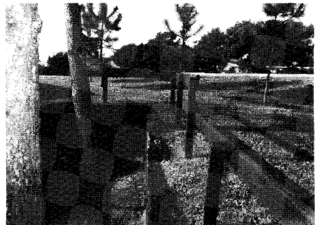
Tree wells can be used to save trees during a grade change.
